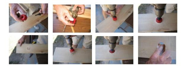
When using a hole saw start with the center drill bit at your center point and drill half way through the board. Then turn the board over and place the center bit in the hole from the other side and finish drilling through the board. Once that's done, sand the hole smooth with sandpaper.
