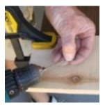
that the door will swing freely. With all parts in alignment pre-drill the two holes for the pivot nails and put them in.
