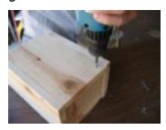
place. Pre-drill the holes and secure with six screws, each placed about 1 1/4" from the edges of the house, two from the front, two from the back and two from the
